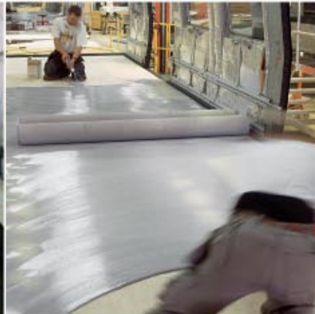
PVC floor bonding with 70-07A
