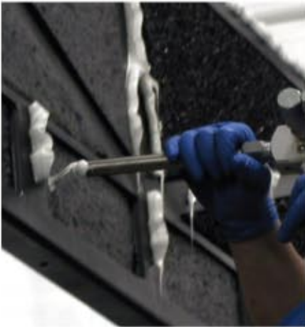
Seam sealing using 2100 SPS
